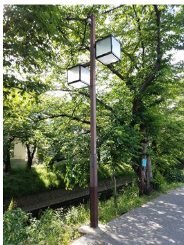
LED照明灯取替
